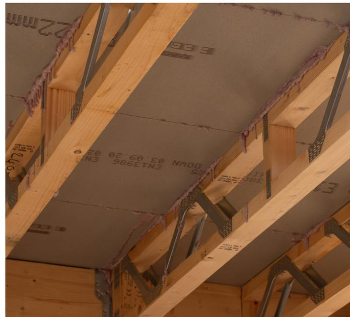
It is essential that the boards are fitted correctly to the joist, the joint is secure (bead of adhesive in the groove and shoulder of the tongue), and that glue is forced up and out of the top surface joint (shoulder of the tongue). The bead of glue applied in the groove of the board will firmly hold the joint in place and will expand out below the joint to protect the underside of the board from moisture ingress.
