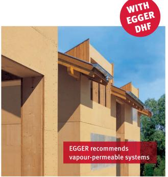
EGGER DHF boards are vapour-permeable wood fibre boards for the external sheathing of **roofs and walls**.
