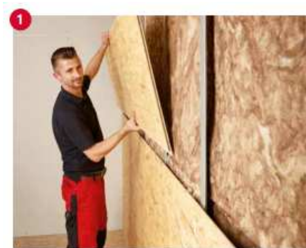
(Image 10): Insert the Ergo Board with the step fold on the long side. To ensure that the various edge profiles are in the correct position, the marking on the surface must be legible from left to right.
