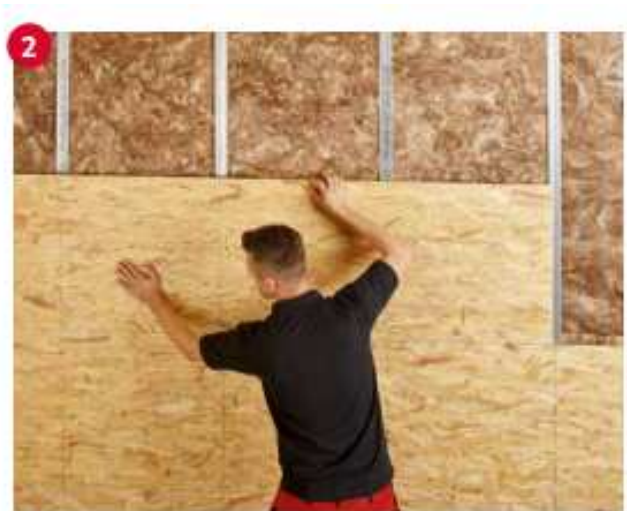
(Image 11): Slide the plate into the correct position, the tongue and groove on the short side interlock with each other.
