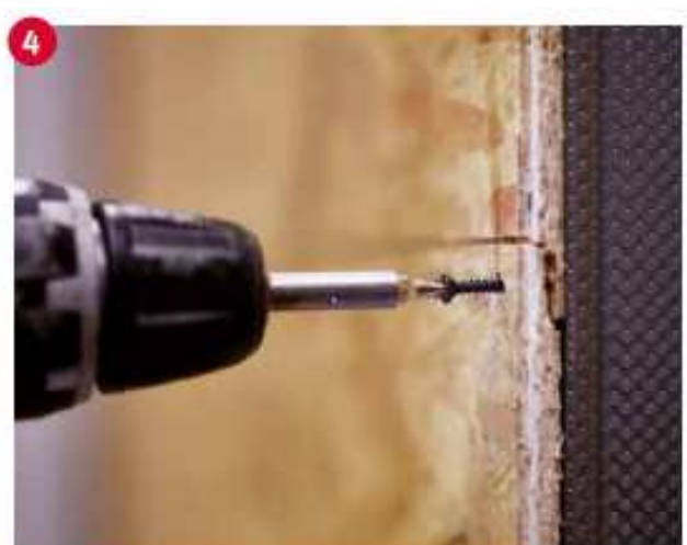
(Image 13): Fastening of the horizontal joints in the stand with a screw. The fastening distance at the edge of the panel is 150 mm, in the center of the panel 300 mm.
