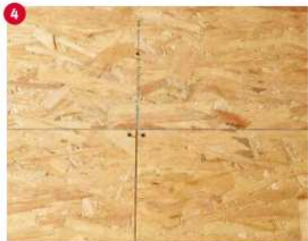
(Image 8): Install the Ergo Board with staggered T-joints.
