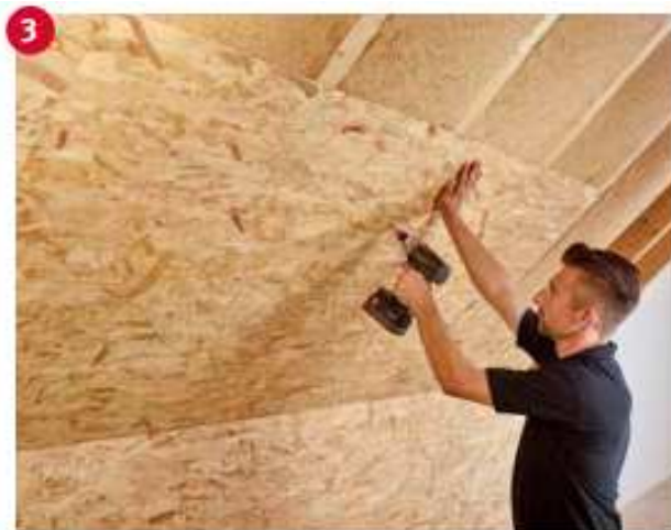
(Image 7): Attach the Ergo Board. It is held securely in position by the edge profiling.
