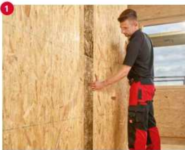
(Image 15): Align the Ergo Board vertically.
