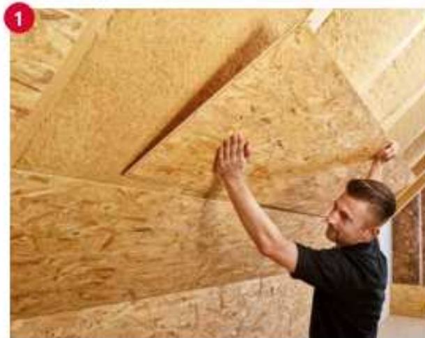
(Image 5): Insert the Ergo Board with the step fold on the long side. To ensure that the various edge profiles are in the correct position, the marking on the top side must be legible from left to right.
