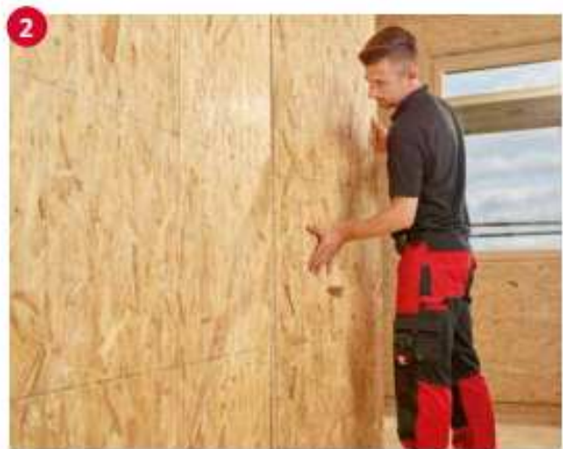
(Image 16): Slide the step seam profiles into each other. The second panel is now held in position.
