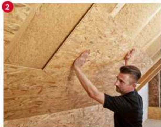
(Image 6): Use the nail grid to find the correct position.
