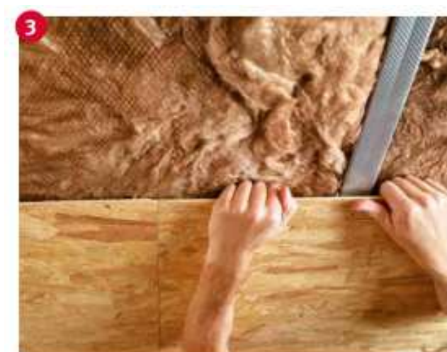
(Image 12): A stable connection is also provided at non-backed panel joints by the tongue-and-groove profile.
