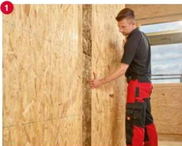
1 Align the Ergo Board vertically.
