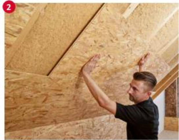
2 Use the nail grid to find the correct position.
