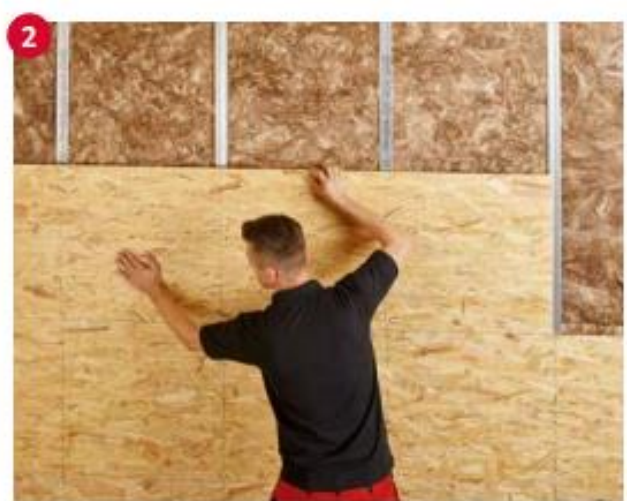
Slide the plate into the correct position, the tongue and groove on the short side interlock with each other.
