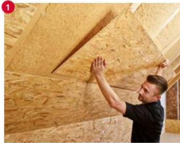
1 Insert the Ergo Board with the step fold on the long side. To ensure that the various edge profiles are in the correct position, the marking on the top side must be legible from left to right.
