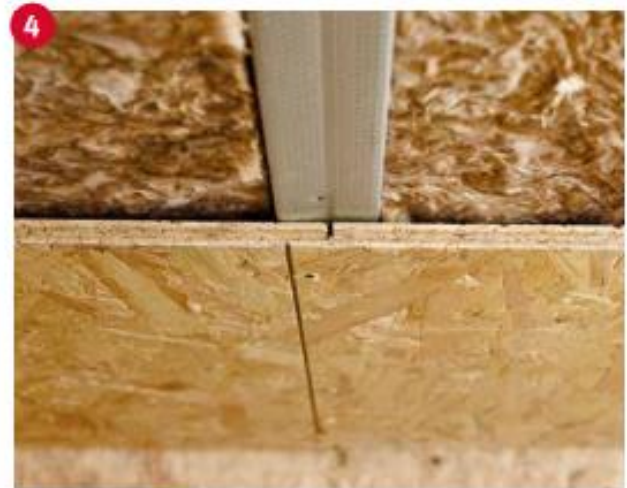
4 Fasten the upright interlocked Ergo Board panels in the step seam area with a screw into the stud frame.
