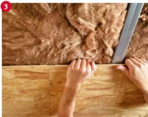
A stable connection is also provided at non-backed panel joints by the tongue-and-groove profile.
