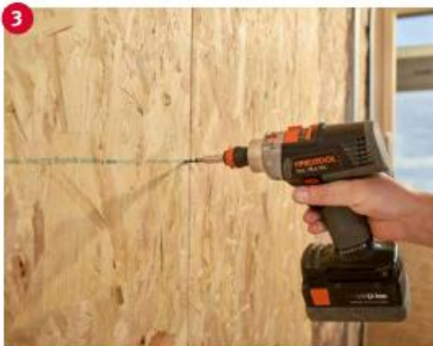
3 Fasten the first Ergo Board with a fastener spacing of 150 mm.
