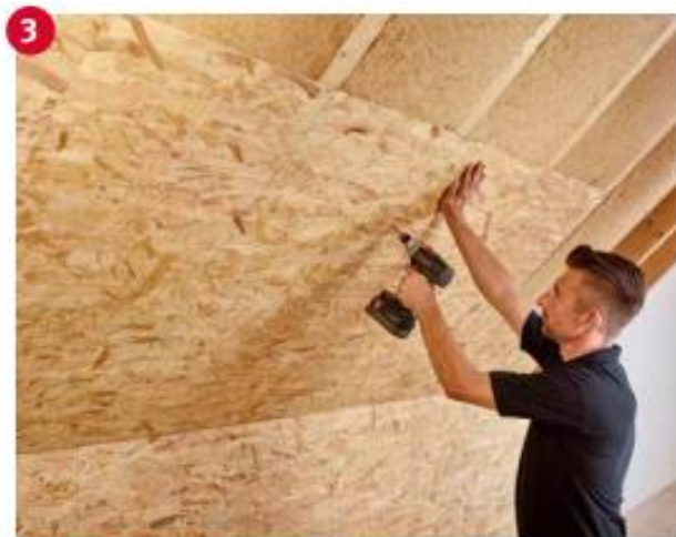
3 Attach the Ergo Board. It is held securely in position by the edge profiling.
