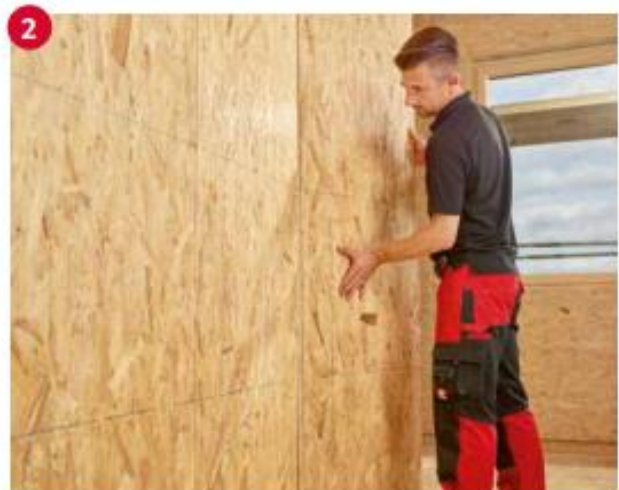
2 Slide the step seam profiles into each other. The second panel is now held in position.
