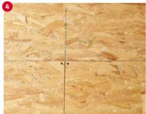
4 Install the Ergo Board with staggered T-joints.
