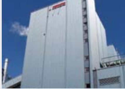
BRILON , since 1991, extension 1993 and 1996. Combustion heat performance: 150 MW Steam performance: 165 t/h
