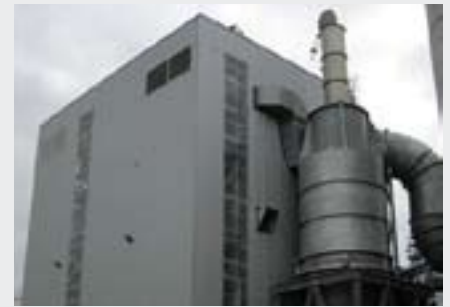
RION , since September 2008. Combustion heat performance: 50 MW 12 MW thermal oil and 38 MW hot gas current
